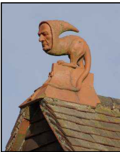
Figure 28 - Terracotta "Gladstone gargoyle" on the roof of The Limes in Penn, Buckinghamshire. Originally sited on the roof of 'Rayners'.
