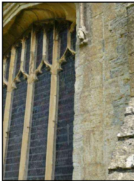
Figure 15 - Female head terminating a drip hood on St Edward's Stow on the Wold.
